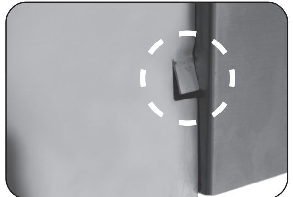
Fig. 25-3 Tab slightly bent in for clearance
